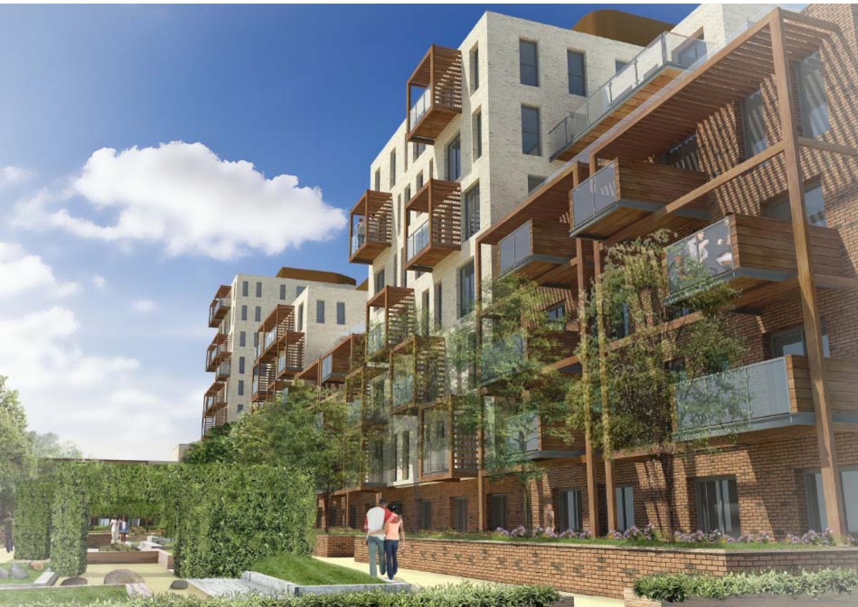
View within central courtyard
